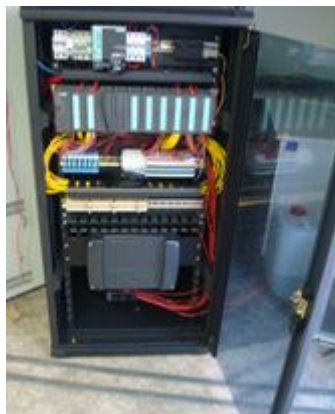
Figure 5: Local permanent – fixed station with fully integrated industrial PLC-based system
