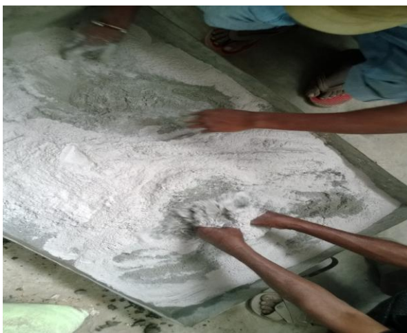
Fig.5 Mixing of cement with RHA
