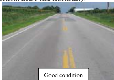
Fig-1: Good condition pavement surface
