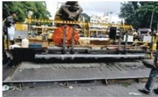
Fig-4: Paver machine in operation
