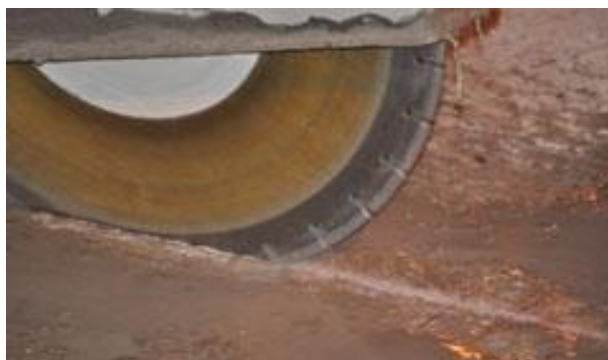
Fig-7: Groove cutting in progress
