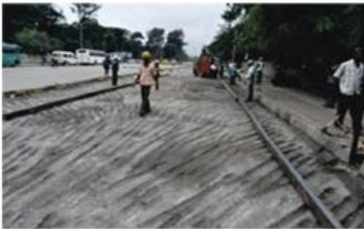
Fig-3: Surface preparation
