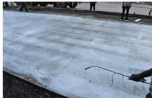
Fig-6: Spraying of curing compound on fresh concrete
