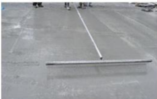
Fig-5: Surface texturing action on green concrete
