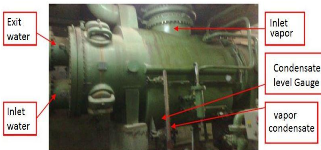
Figure 1. Condenser setup in industry
