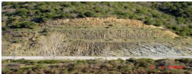
Photo 2: Characteristic folded structure along the existing road
