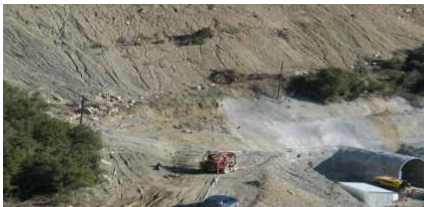
Photo 4: Drainage tunnel 1A.
