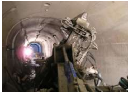
Photo 8: Drilling drainage holes in the drainage tunnel.
