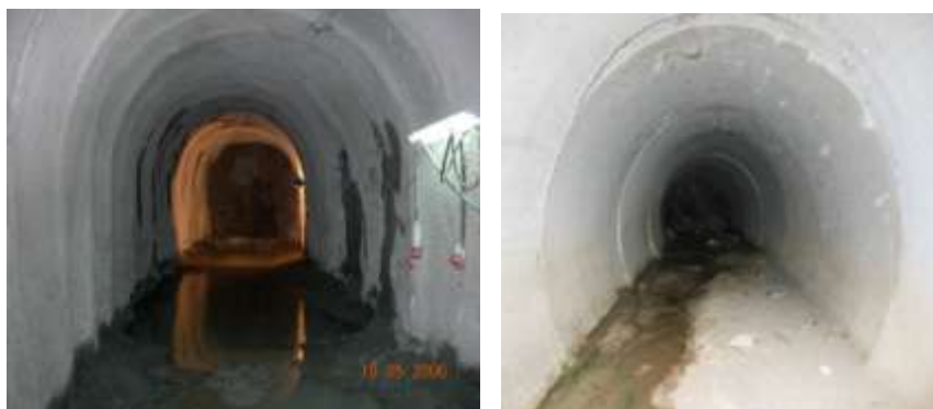
Photos 5 and 6: Drainage Tunnel 1A (before and after the final coating).
