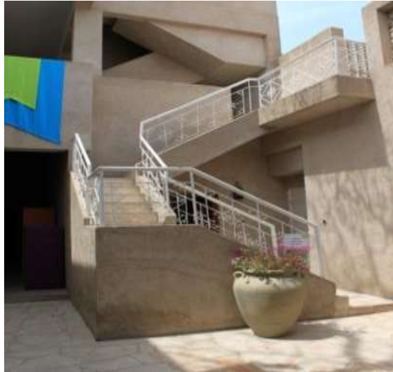
The staircase handrail which is added does not reflect the sense of historical place.
