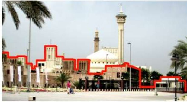
Skyline where the wind towers are part of the composition.
