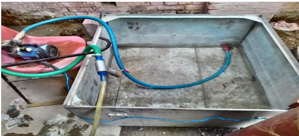
Fig 5- Water tank for hot water and cold water restore
