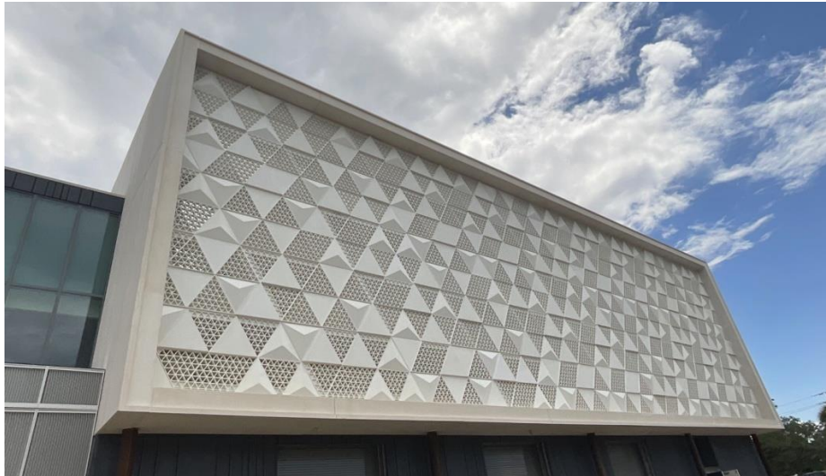
Figure 3. Baptist Health Regional Hospital Façade using Non-Metallic Fiber UHPC
