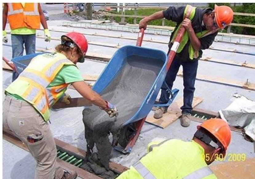
Figure 2. Connection Link Between Precast Elements
