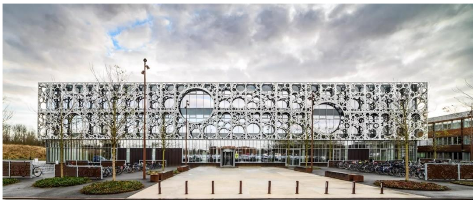
Figure 4. The University of Southern Denmark - UHPC Façade
