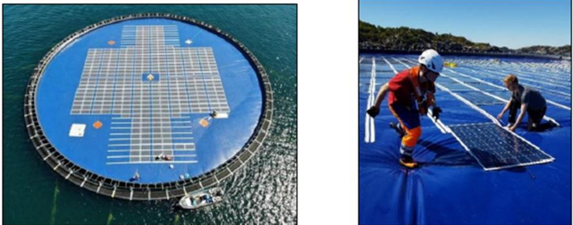
Figures 7 and 8: Membrane floats and mats. Source: Ocean Sun (2019).
