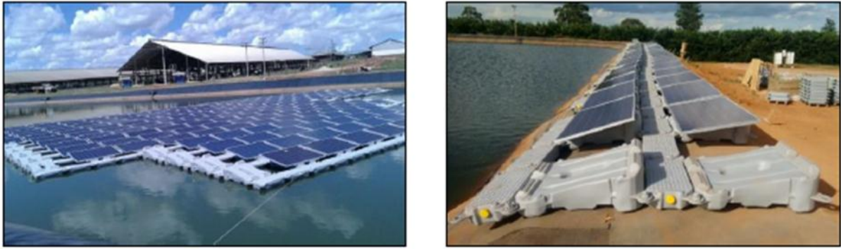
Figures 03 and 04: Direct module attachment type floats. Source: Sunlution (2019).
