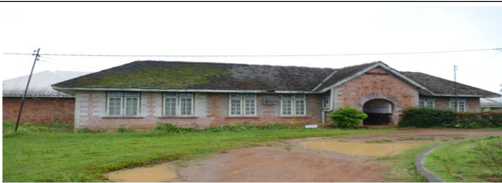
Figure 7: ENIEG Kumba Administrative Building
