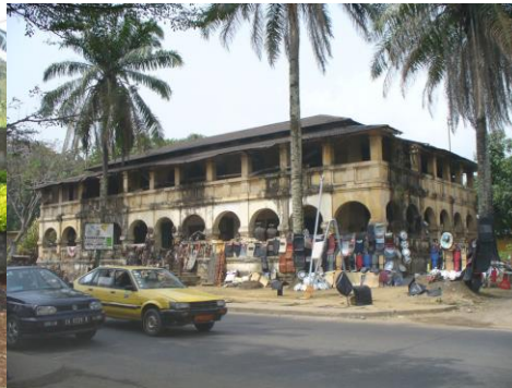
Figure 6: Old German building in Dja (Villa Mandessi Bell)
