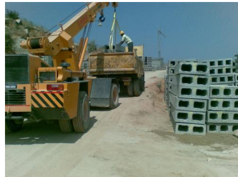
Figure-4: Lifting of RCC columns
