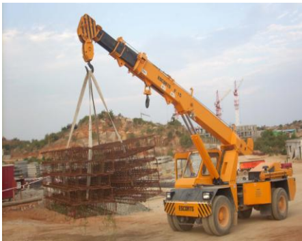
Figure-3: Conveyance of steel frames RCC columns
